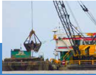
Proyek | Project Dredging & Lifting Mahakam-East Kalimantan
