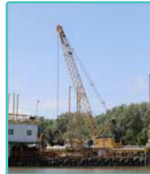
Sanga - Sanga Site Office Kalimantan Timur East Kalimantan
